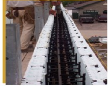
3. Place Rebar In The Walls
