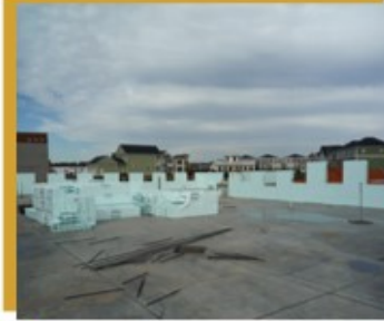
2 Stack Forms & Create Openings
