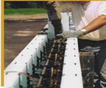
5.Pour Concrete Into Walls
